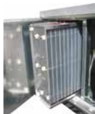
Electrostatic filters 0,01\mu\text{m} > x > 10\mu\text{m}
