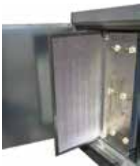
Aerosol panel filters x > 100\mu\text{m}
